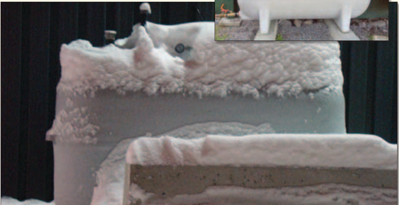
Top: Fibreglass heating oil tank on concrete stands. Bottom: Fibreglass heating oil tank. Note the concrete barrier protecting the tank.
