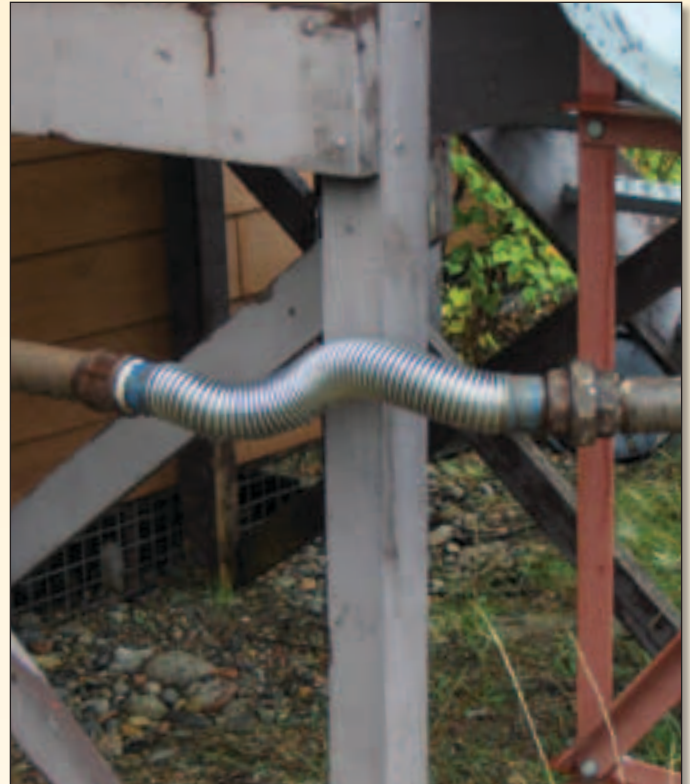
This flex connector is out of alignment.
