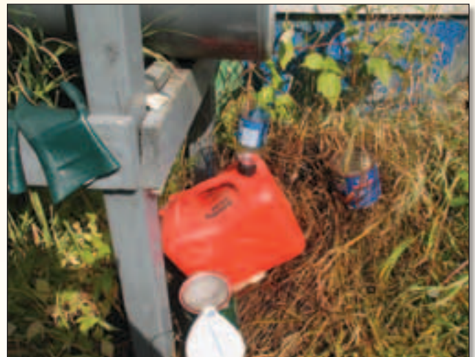
Attempt to capture oil leak. Note the dead vegetation around the tank.
